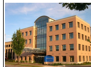
Summit Place Industrial to Office Space Adaptive Reuse (West Allis, WI)
